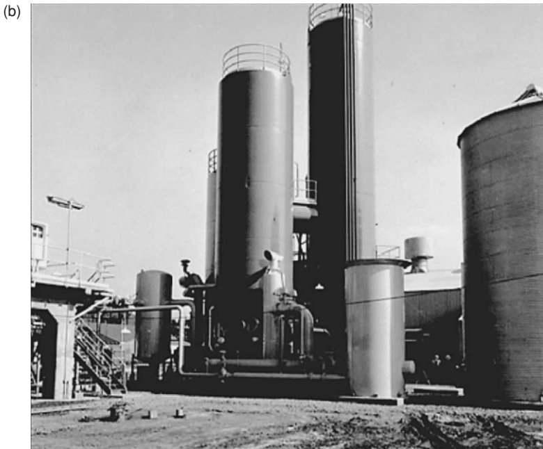
FIGURE 1.16. (a) 2 ton/day oxygen plant available around 1910. (b) 100 ton/day oxygen plant available in the early 1950s.
