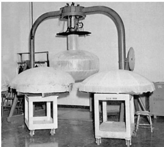
FIGURE 11.7. Early testing by Lockheed of candidate constructions of MLI.
