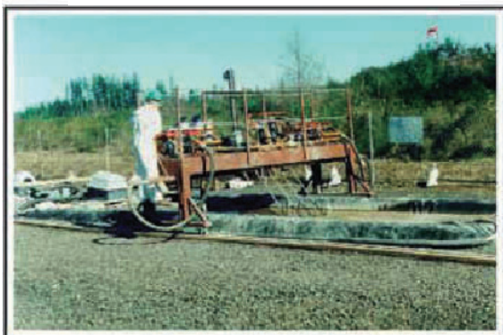
40 Cubic Yard Demonstration
