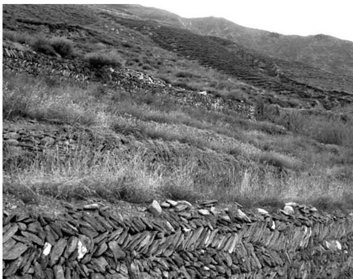
FIGURE 50.1. Rock terraces constructed in Sichuan Province, China to reduce runoff and soil erosion during the establishment of trees. The availability of labour and the local presence of rocks made this scheme possible in this situation. (Photo © Steve Whisenant.)
