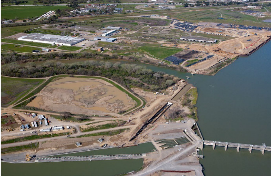
Fig. 7 Red Bluff Diversion Dam and canal [26]
