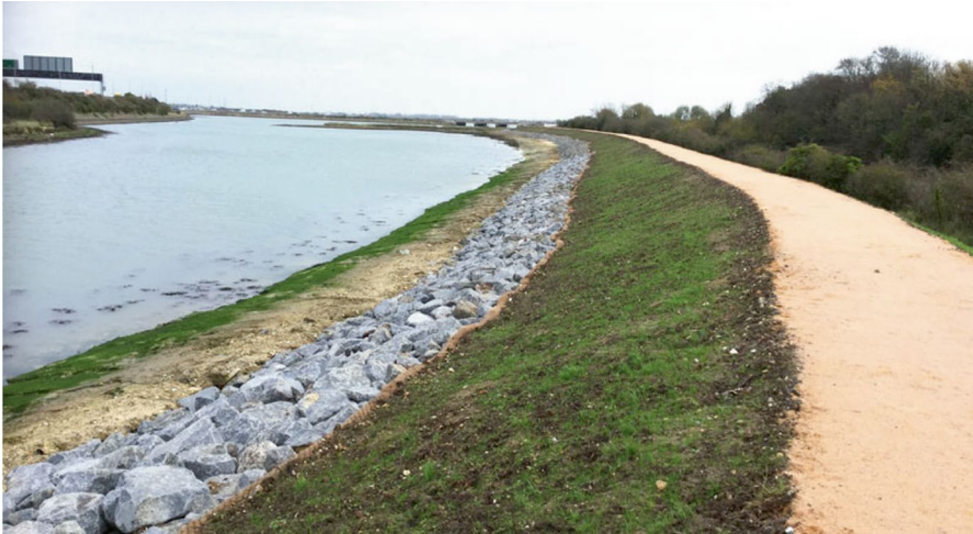
Fig. 9 Levee Portsea Island [30]
