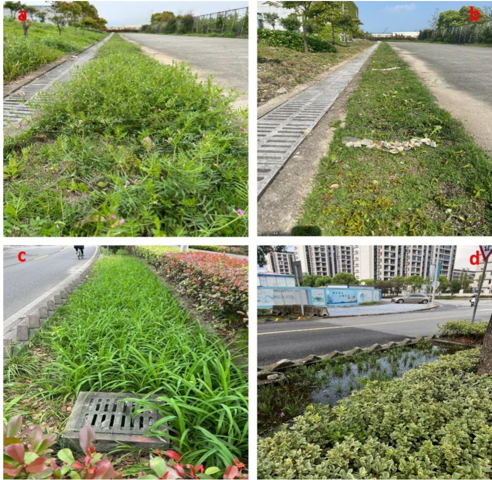
Fig. 3 Four types of green swales were constructed in different areas, including (a) grass swales, (b) infiltration swales, (c) bioswales, and (d) wet swales.
