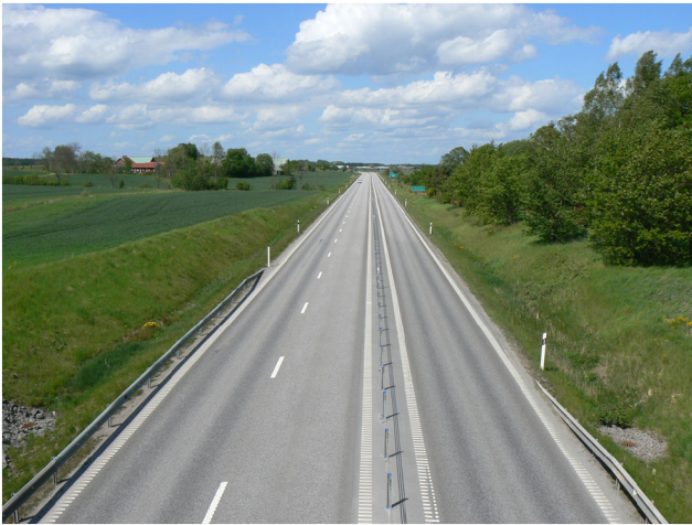
Fig. 1 An example of a 2 + 1 road with cable barriers in Sweden (Wikipedia contributors. “2 + 1 road.” Wikipedia, The Free Encyclopedia. https://en.wikipedia.org/w/index.php?title=2%2B1_road&oldid=741622137 . Accessed on November 7, 2016)
