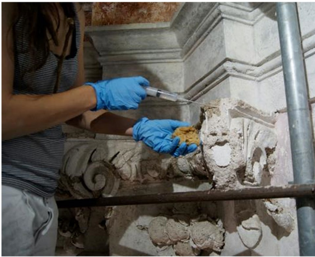
Fig. 6 Consolidation of a disaggregated mortar using Ethyl silicate applied by syringe
