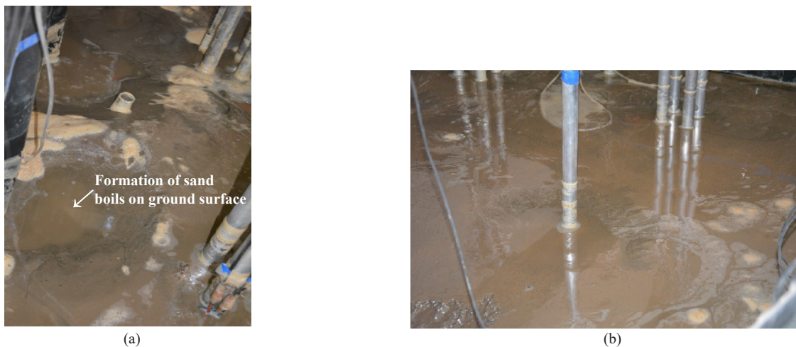
Fig. 11 (a) Formation of cracks on the ground surface through which water rose up to ground surface; (b) formation of cracks/sandboils near the piles
