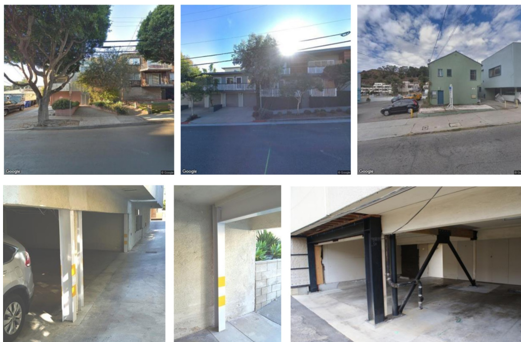
Fig. 10 Problems to be addressed in the future. Top: Example of problem images: occlusions (1st) and multi-buildings (2nd and 3rd). In the 3rd image, the left building is actually a soft-story; however, its opening space is located on the other side of the building. Bottom: Example images of a retrofitted soft-story. As shown in the 3rd image, some reinforced structure is added inside the building, which may not be captured by street view images. The 1st and 2nd images are from the official website of the LA Department of Building and Safety, and the 3rd is from a California Foundation Repair Contractor
