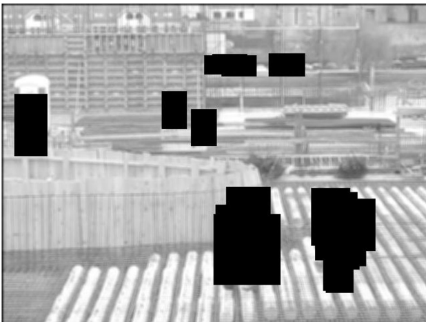
Fig. 6 An example of recognizing and masking the moving objects on a construction site, some of them being workers
